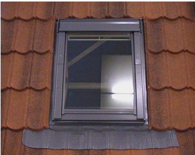
Finished Rooflight
